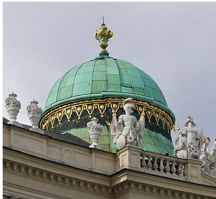
Figure 2: Hofburg Vienna dome with green-colored oxidized copper coating. Picture source: https://commons.wikimedia.org (pictures placed into the public domain).
