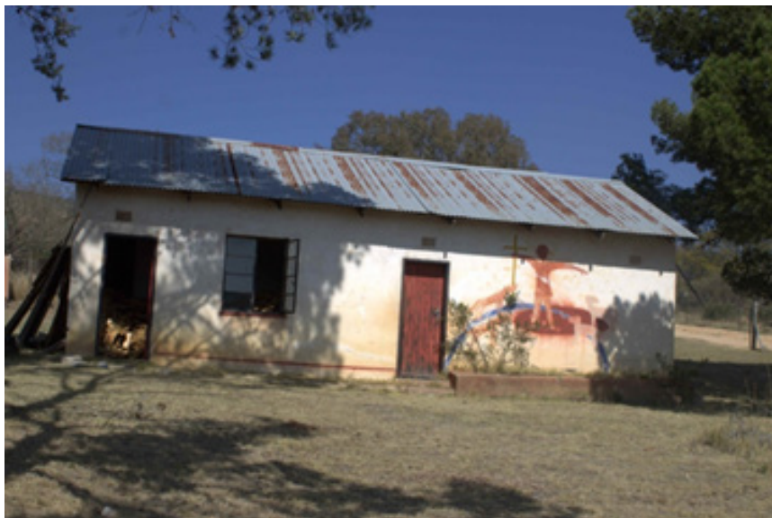
Figure 1: Lutheran Missionary Health centre buildings at Masealama, Mankweng Area.
