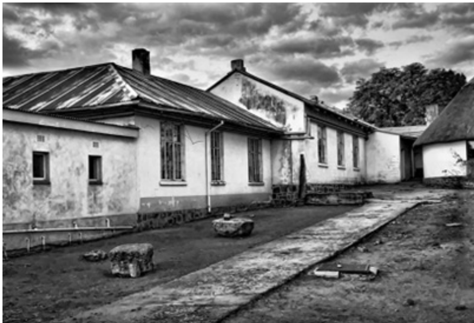
Figure 2: The older buildings of Jane Furse Memorial Hospital.
